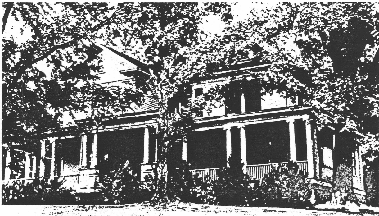
The home of Zachary Taylor Smith in Mount Airy, lost to the developer's bulldozer in 1969
